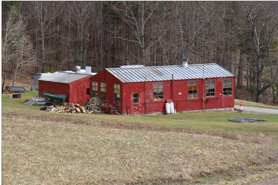
Photo 7.27: A c. 1960 gas compressor station, Greenwood (TRC# 1171) (David Price, April 3, 2017, Image# 1549).
