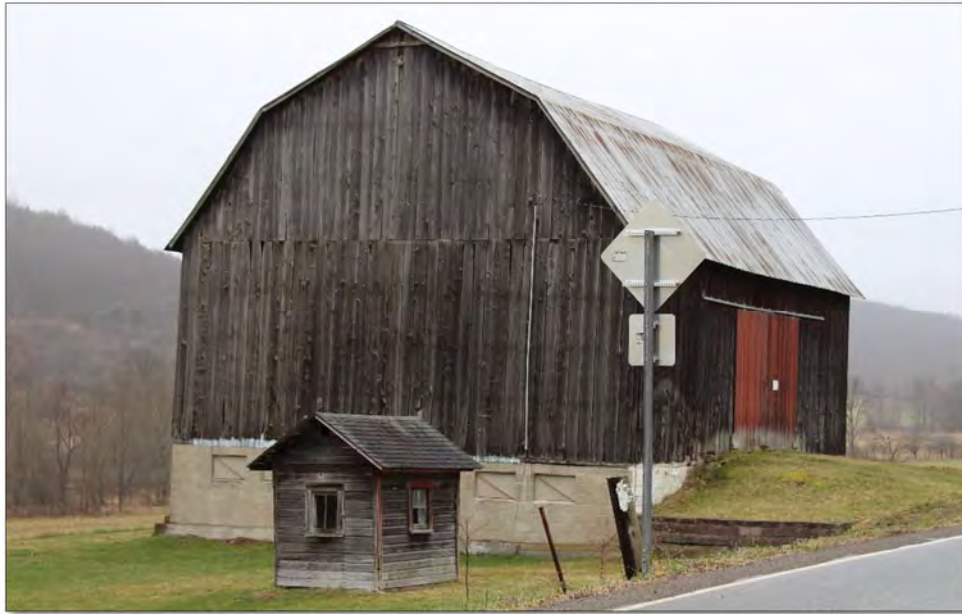
Photo 7.17: Typical late nineteenth- or early twentieth-century side gambrel barn on a high basement. This form is the most common to the survey area (TRC# 1680) (Philip A. Hayden, April 6, 2017, Image# 720).
