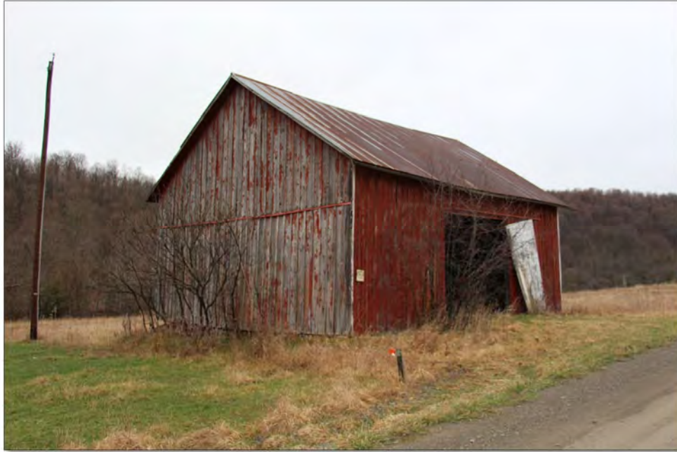
Photo 7.19: Typical mid- to late nineteenth-century side gable barn on ground-level foundation (TRC# 1702) (David Price, April 6, 2017, Image# 1908).
