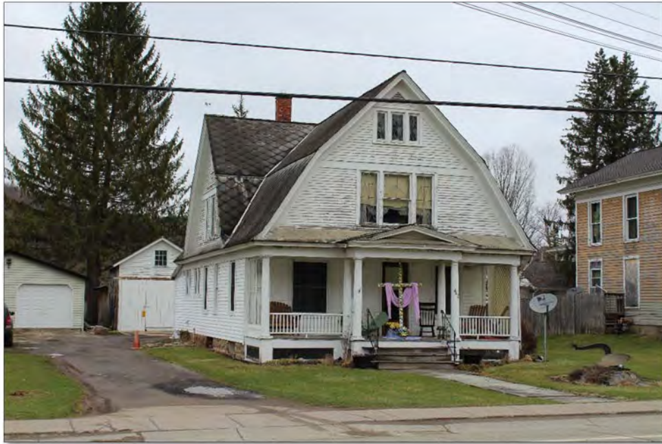
Photo 7.11: Typical Gambrel roof Dutch Colonial Revival-style mail-order residence, Village of Whitesville (TRC# 1499) (Philip A. Hayden, April 5, 2017, Image# 417).
