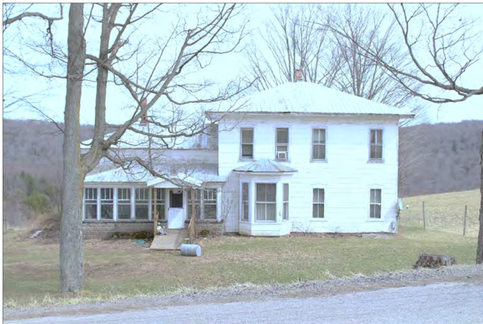
Photo 7.4: Typical vernacular hipped roof Italianate-style farmhouse with wing (TRC# 1751) (Philip A. Hayden April 3, 2017, Image# 185).
