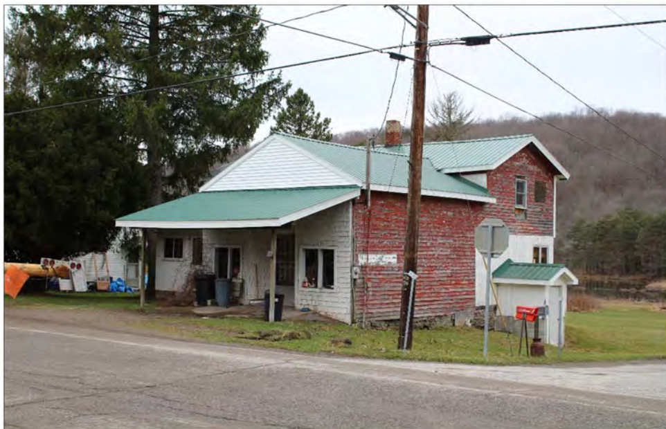
Photo 7.46: View of the intersection of CR 248 and Cemetery Hill Road, Village of Rexville, looking southwest depicting the commercial core (TRC# 1854) (Philip A. Hayden, April 5, 2017, Image# 379).
