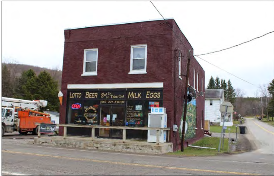
Photo 7.45: View of the intersection of CR 248 and Rexville-Troupsburg Road (Church Street; CR 117), Village of Rexville, looking southeast depicting the commercial core (TRC# 1853) (Philip A. Hayden, April 5, 2017, Image# 380).
