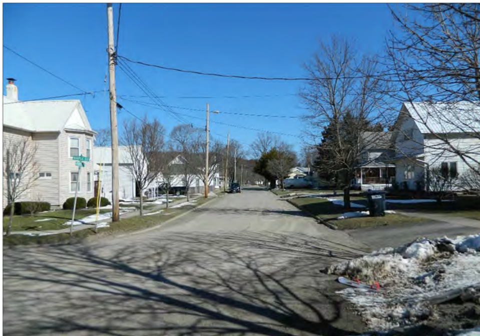
Photo 7.32: View of First Street, Village of Andover, from the intersection of Maple Avenue looking north (Jessica Burr, March 23, 2017, Image# 9669).
