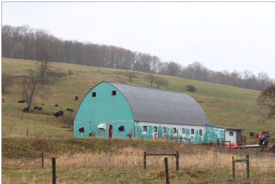
Photo 7.20: A relatively rare example of a twentieth-century Gothic roof barn available through mail-order suppliers (TRC# 1781) (Philip A. Hayden, April 4, 2017, Image# 326).
