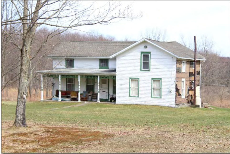
Photo 7.1: This common wood-framed vernacular residence with side wing typified most farmhouses (TRC# 1815) (Philip A. Hayden, April 3, 2017, Image# 204).
