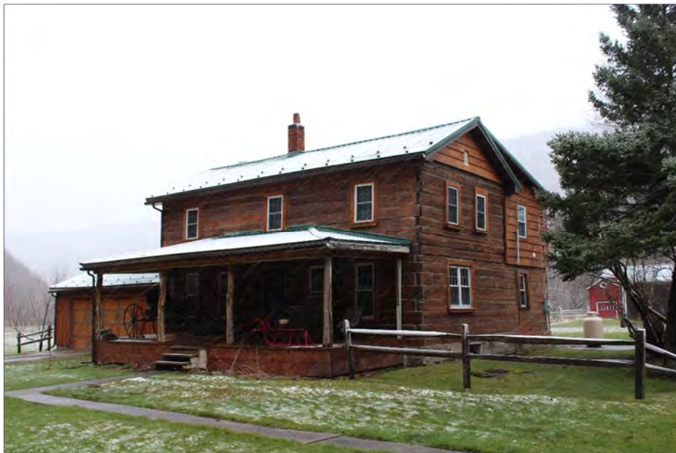
Photo 7.2: This exposed cut log house with false-corner construction comprised the only identified building of log construction (TRC# 1288) (Philip A. Hayden, April 7, 2017, Image# 765).
